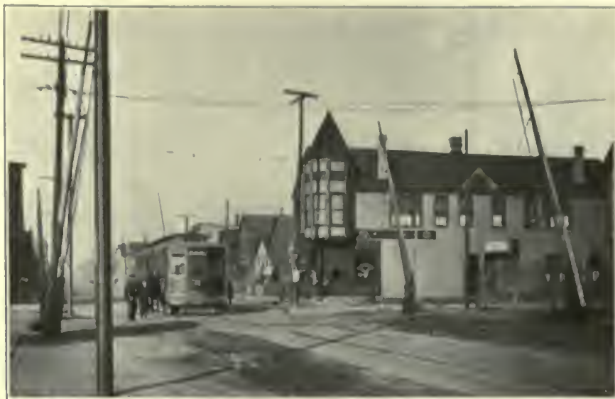
FIG. 249. GRADE CROSSINGS. Highway and electric railway crossing of the Elgin, Joliet & Eastern Railway at 86th Street and Burley Avenue.
